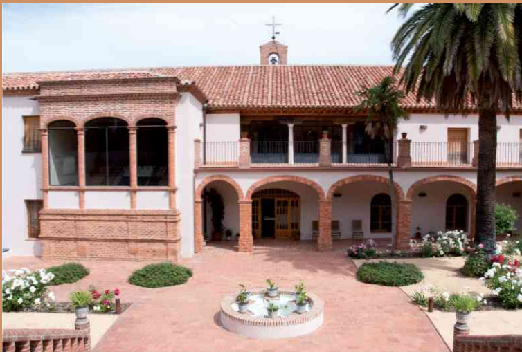
Patio interior del Hospital
